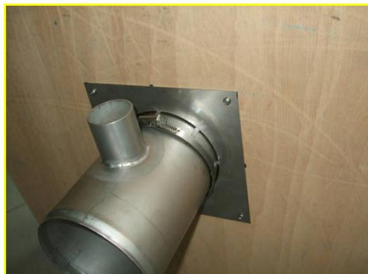
9.) Pull backwards the mixing tube until the limit stop. In the next step pull the hose clamp and the flange plate together until the wall.
